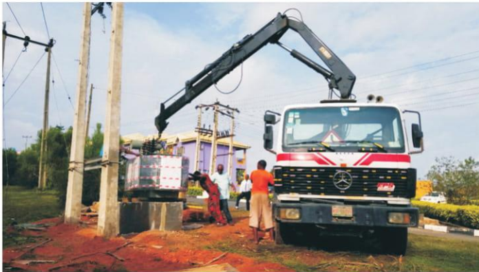
Installation of 33 KVA transformer to the university for better power supply
